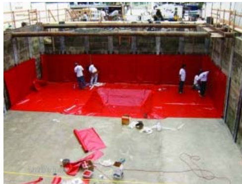
At the Assael Residence, Ekedal Concrete sandwiched the waterproofing membrane in between concrete slabs to prevent rebar from puncturing it.
