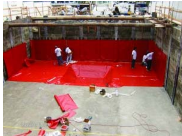
At the Assael Residence, Ekedal Concrete sandwiched the waterproofing membrane in between concrete slabs to prevent rebar from puncturing it.
