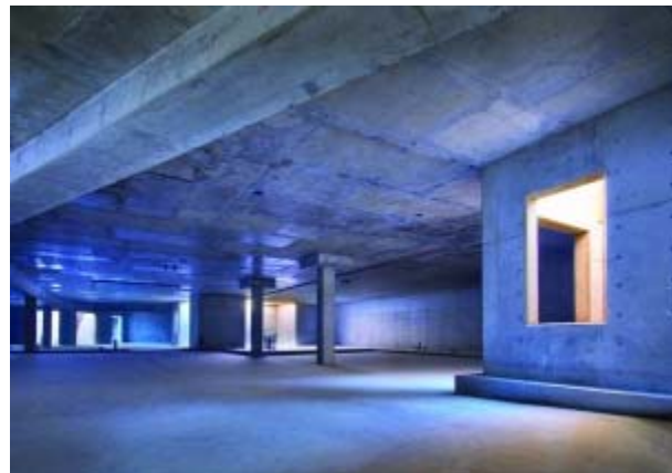
At the Assael Residence, Ekedal Concrete sandwiched the waterproofing membrane in between concrete slabs to prevent rebar from puncturing it.
